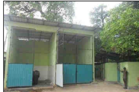
Figure 2 - Waste storage & bins at Lady Ridgway Hospital
